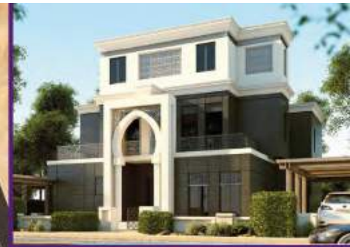
GAWHARET ELASAMA Client: Engineering Authority of Armed Forces. Location: New Capital, Egypt.
